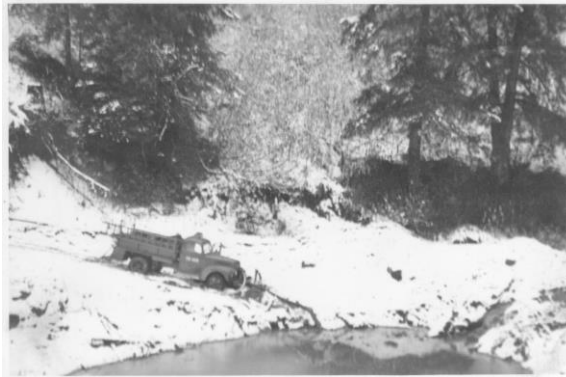
Fire truck pumping.....near MP 48
