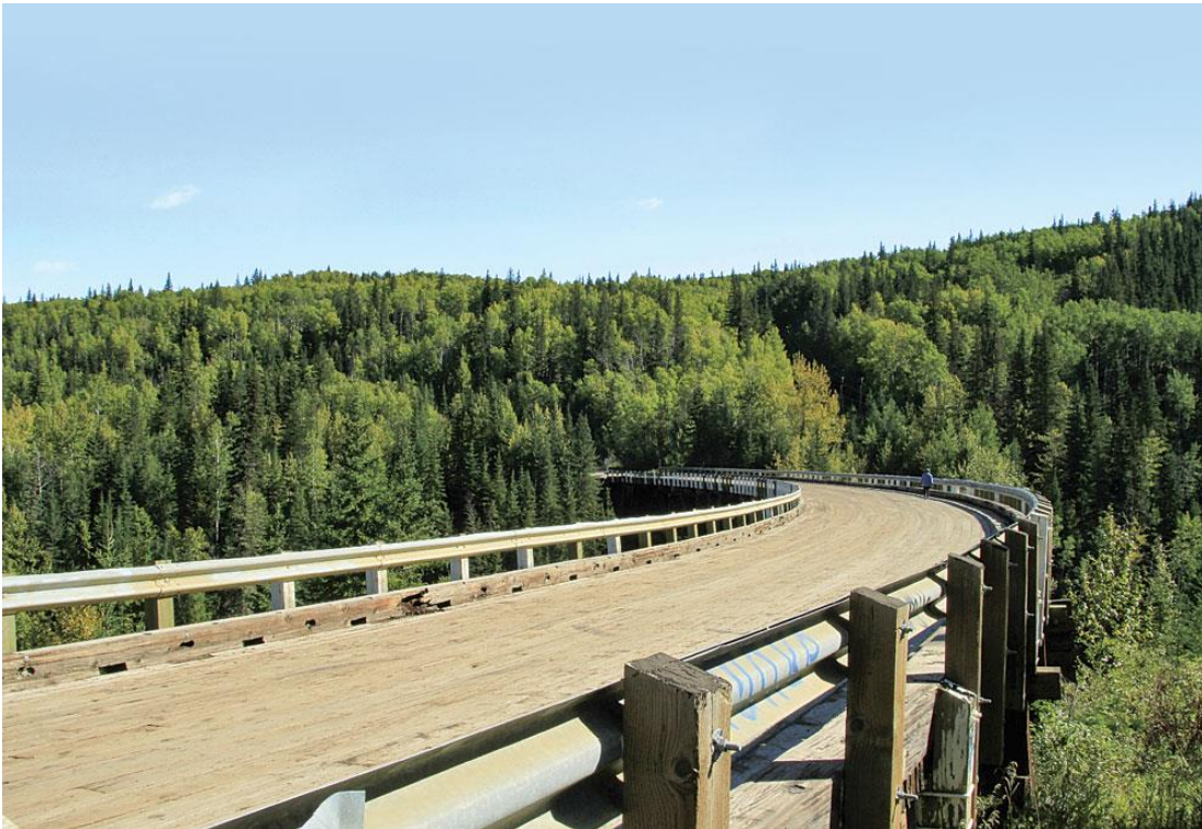
Curving 9 degrees along its 534-foot timber span, the Kiskatinaw Bridge is the only original Alaska Highway bridge still in use.
