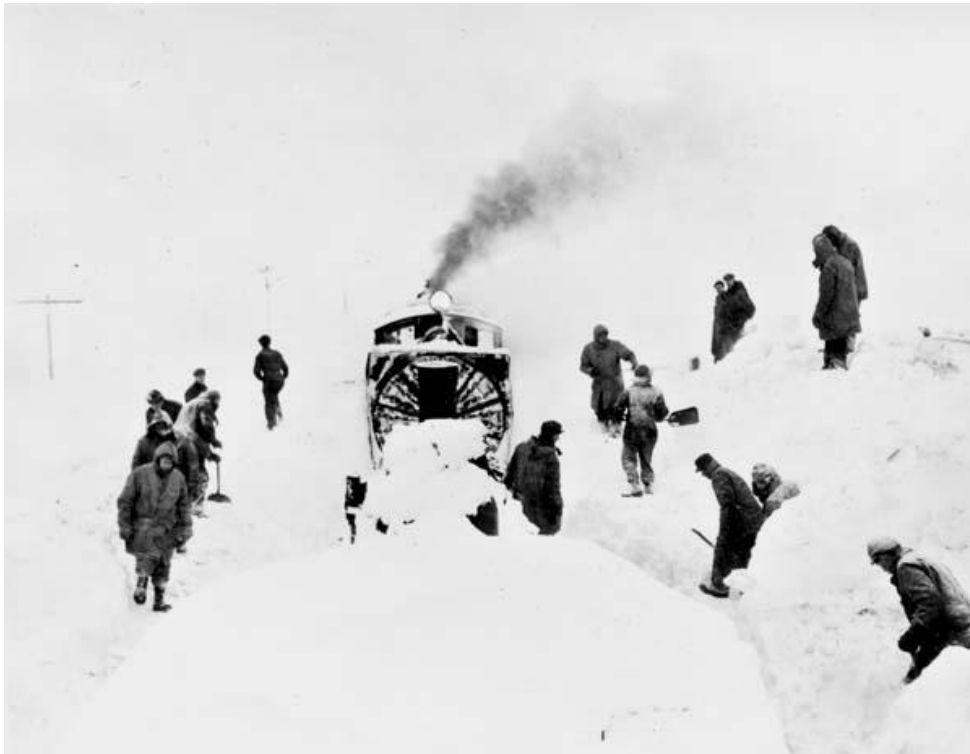
Snow plows and crews digging out a snowbound train. W.P. & Y.R. White Pass Rotary rescuing snowbound train Mile 16-17 on RR. Yukon Archives. William J. Preston fonds, #15.
