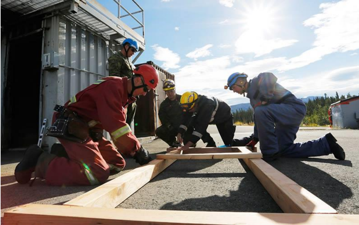
Participants create stabilizing beams during an urban search and rescue training course Tuesday.
