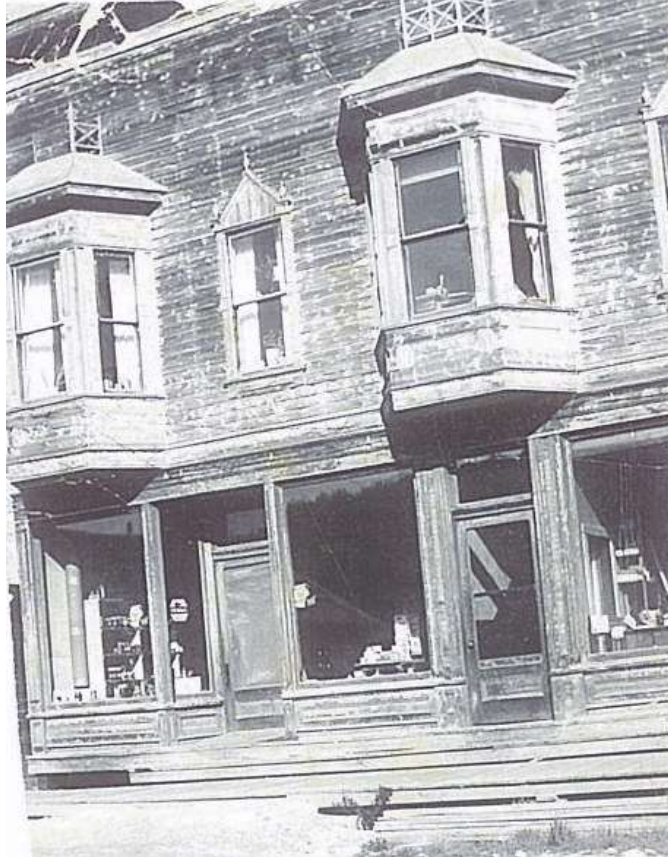
Caley's General Store, Third Avenue, Dawson, is noteworthy for its false front, large shop windows and the cantilevered box bay windows on the second floor. (Photo courtesy of Caley family).
