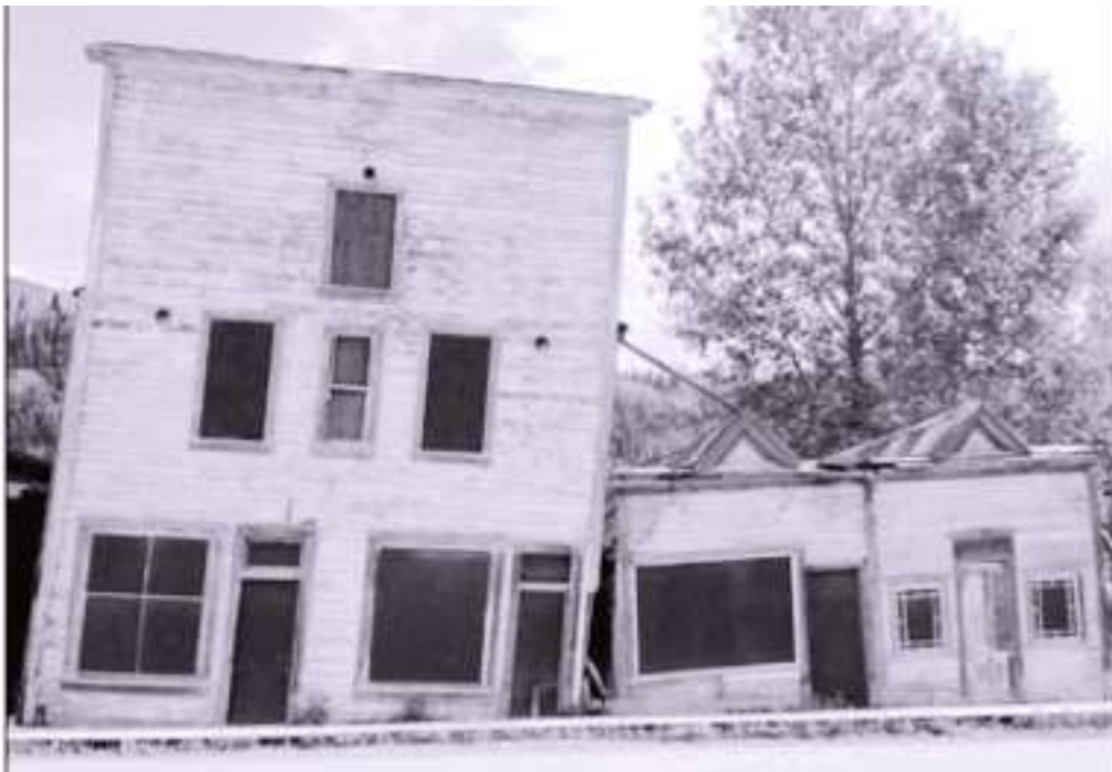
The permafrost-ravaged Ellingsen Store Complex, Third Avenue, between Princess and Harper streets, was built in 1901 and bought in 1912 by Erling Olav Ellingsen for his photography studio and the Minto Hotel. (Klondike Sun Photo by Thomas Seibel, 2008)
