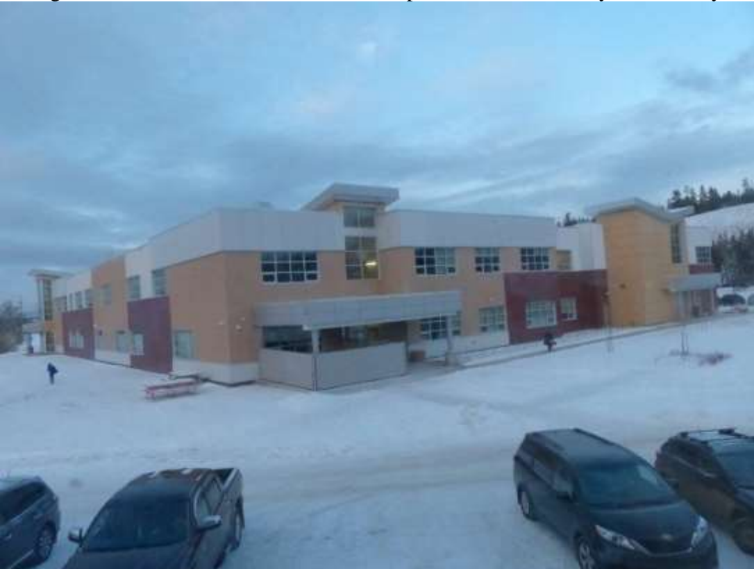
New FH Collins School as seen from old school.
