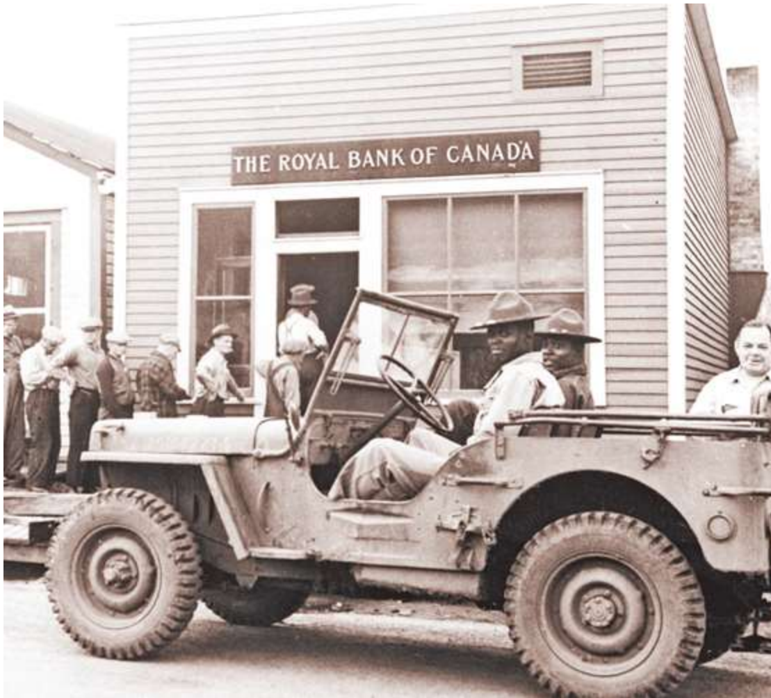
Bechtel employees and U.S. Army soldiers wait outside a bank in Fort McMurray, Alta., on payday during preparations to supply the Canol camp in August 1942.
