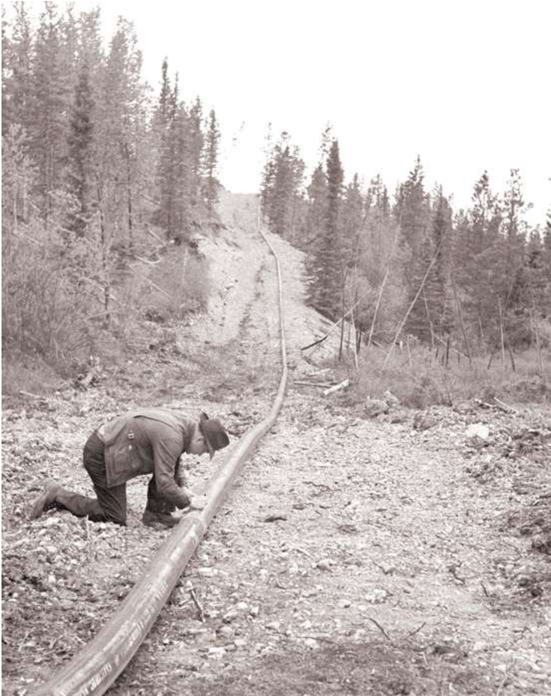
An oilman checks the welding on a section of the pipeline in June 1943. HARRY ROWED/NFB/LAC/PA-174542
