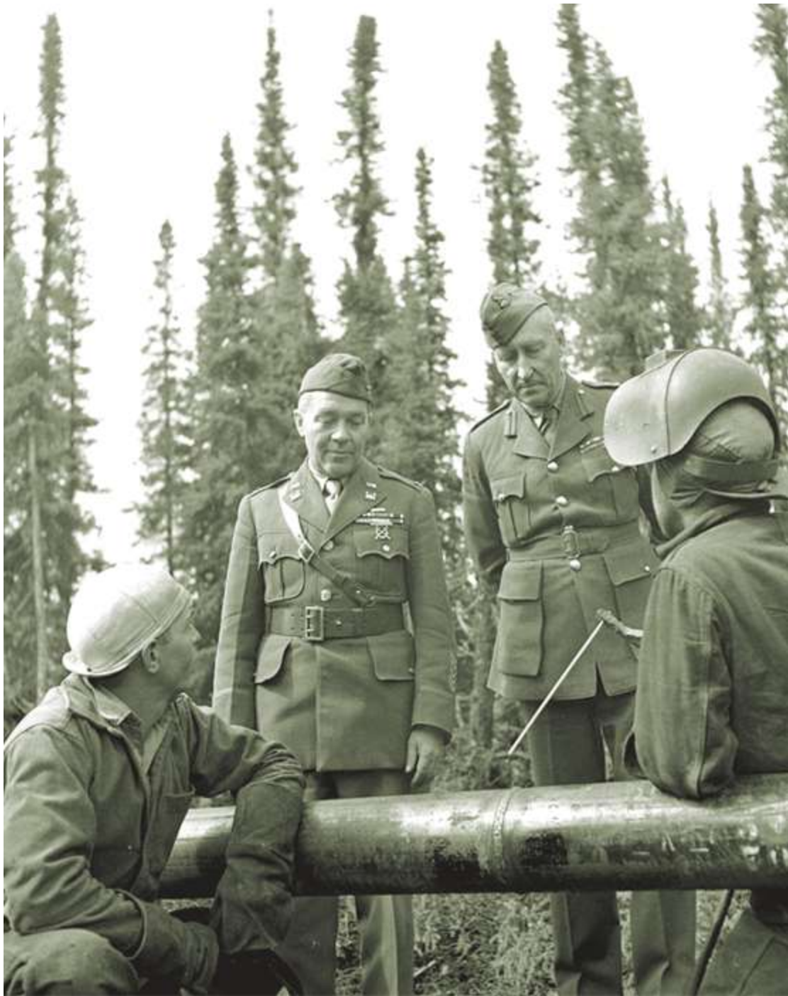
Major-General W.W. Foster of the Canadian Army (below, at right) and his aide chat with workers on the pipeline in June 1943.
