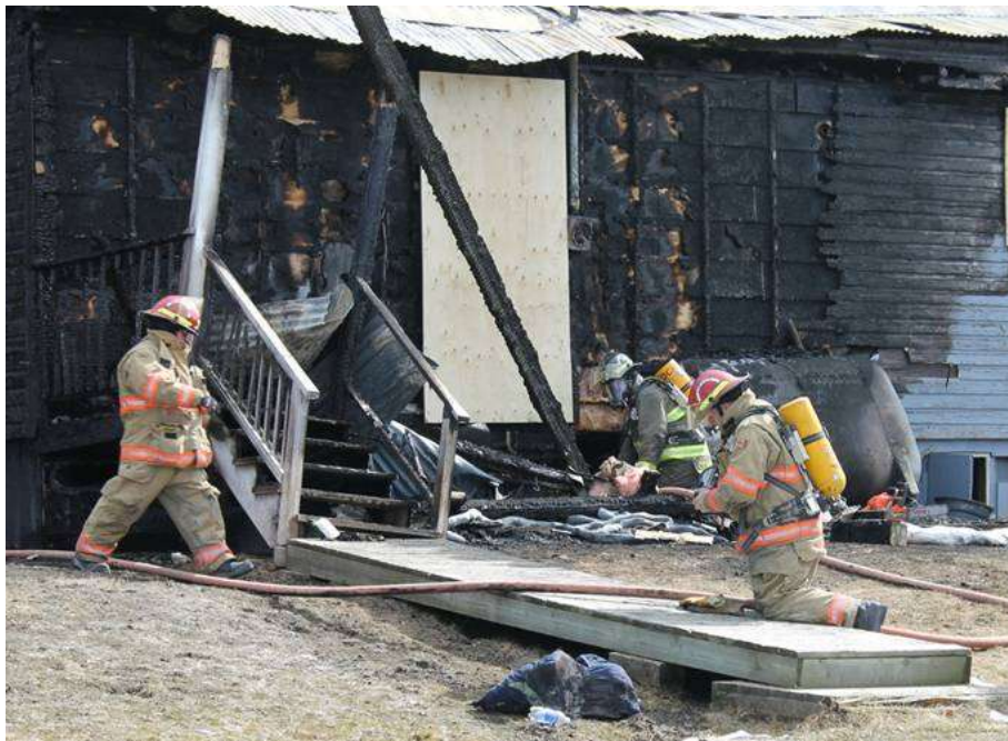
The smoldering was in the crawlspace on the west side of the building. Photo courtesy Dan Davidson uffish@northwestel.net (In Dawson)
