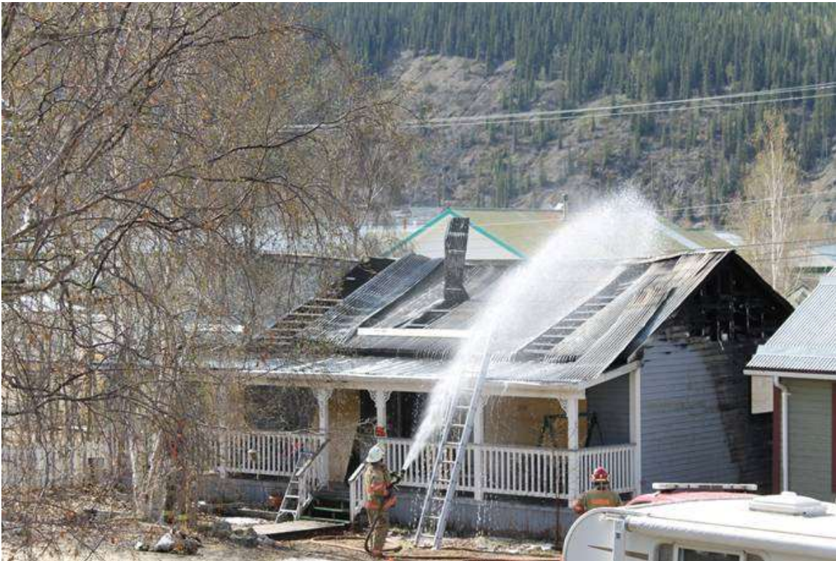
Spraying down the outer roof to get to the original roof area. Photo courtesy Dan Davidson uffish*northwestel.net (In Dawson)
