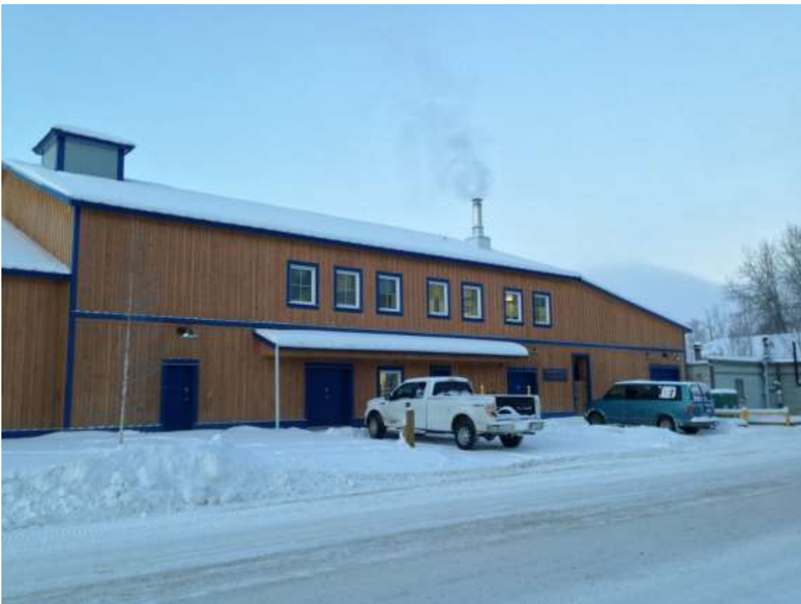
Waste Water Treatment Plant – Dawson hasn't taken ownership of this plant yet – and doesn't want to until it works properly.
