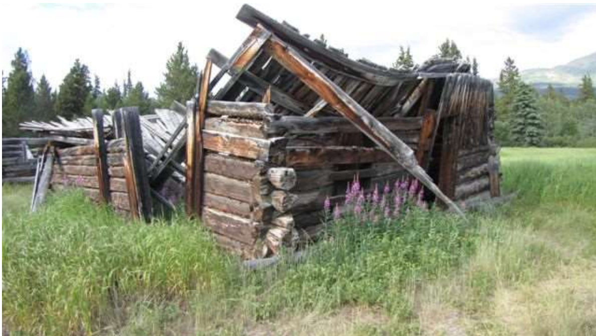
Robinson Roadhouse buildings
