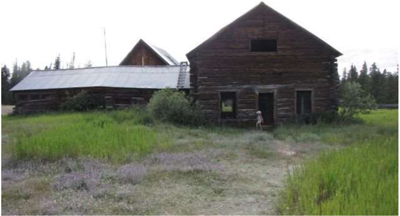
Robinson Roadhouse buildings
