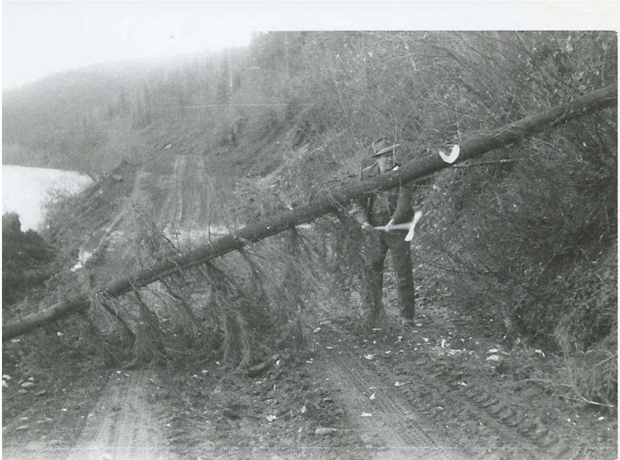
Klondike Highway near Asbestos bluff 1953. John Gould photo.
