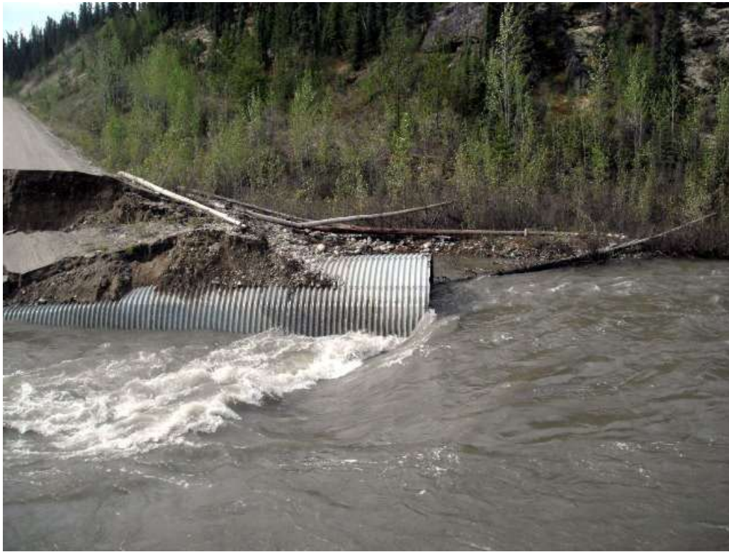
Conglomerate Creek 2 Photo courtesy Al Gladda, foreman at North American Tunsten.
