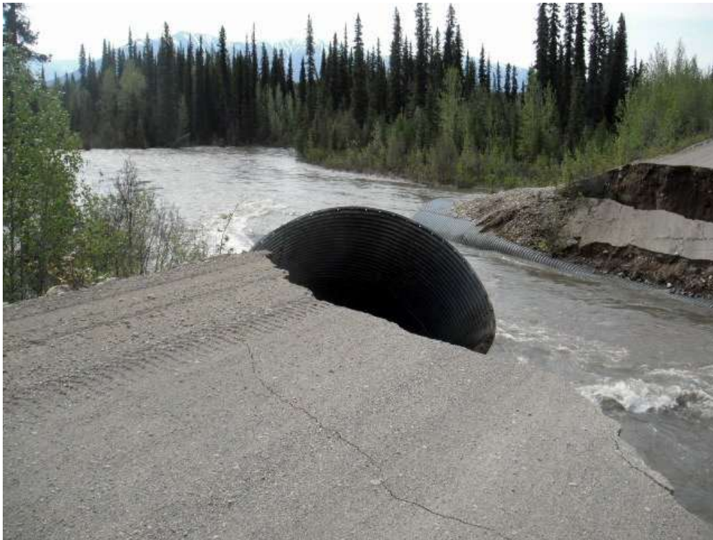
Conglomerate Creek Photo courtesy Al Gladda, foreman at North American Tunsten.
