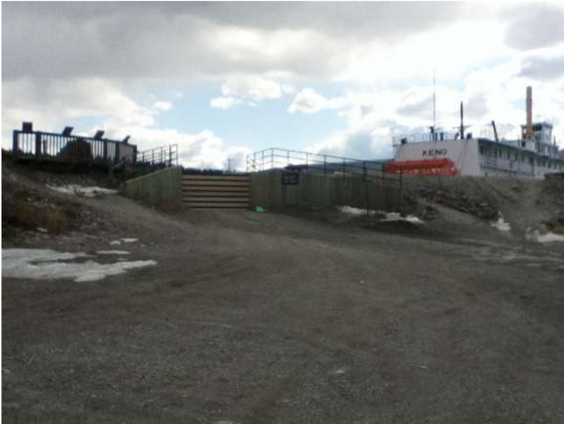
Wooden and steel barrier that blocks the hole in the dyke in Dawson. Photo courtesy Dan Davidson uffish*northwestel.net (In Dawson)
