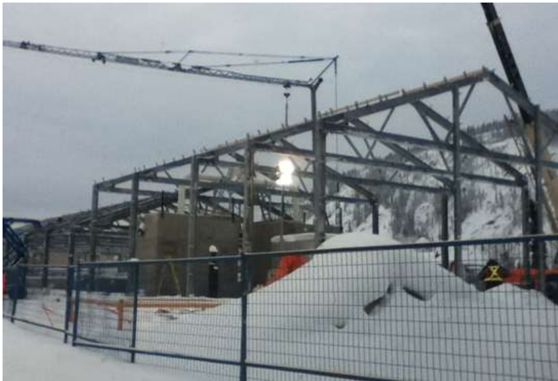
Roof Trusses installed Photo courtesy Dan Davidson uffish@northwestel.net (In Dawson)
