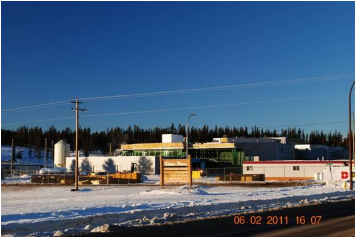
New Jail under construction, over budget. Photo courtesy Grant Lundy waterquality*klondiker.com (In Whitehorse)
