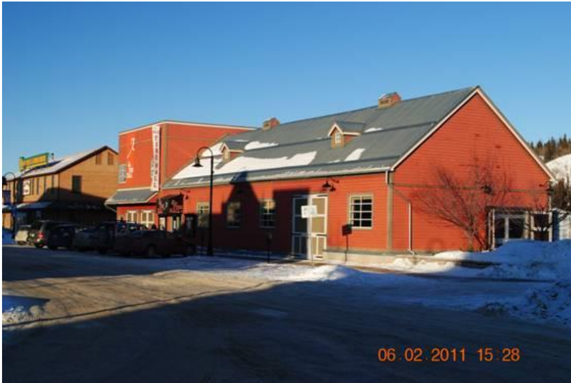
New Old Fire Hall
