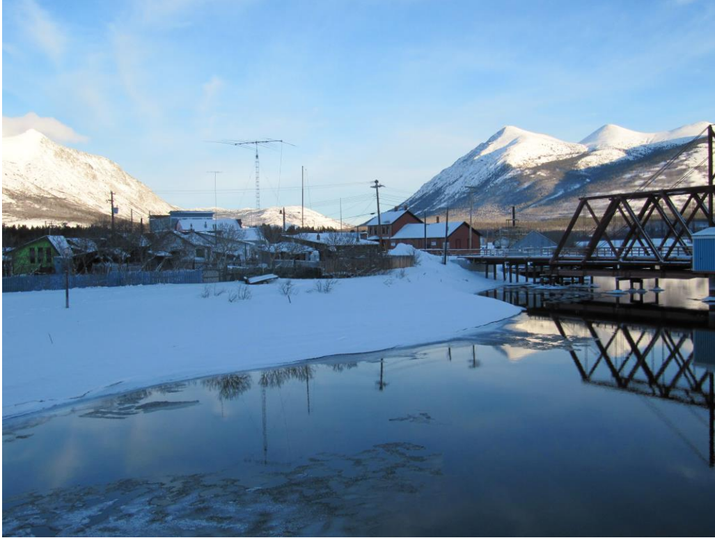
White Pass bridge and station Jan 1, 2011
