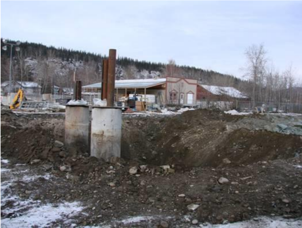
The coffin was found while excavating around these twin shafts, the heart of the Corix Water Systems' VERTREAT (VERTical TREATment) system. Photo courtesy Dan Davidson uffish@northwestel.net (In Dawson)
