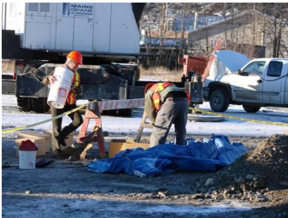
These tarpaulins protected some of the excavated dirt in which the bones were discovered. Photo courtesy Dan Davidson uffish@northwestel.net (In Dawson)
