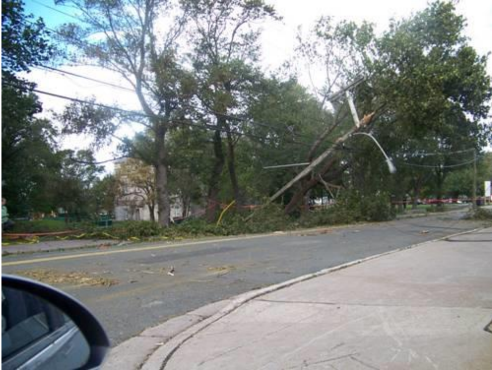
A power pole lost out to the weight of a tree which was up rooted. Photo courtesy Gus Barrett sourdoughs2@shaw.ca (In Qualicum Beach BC)
