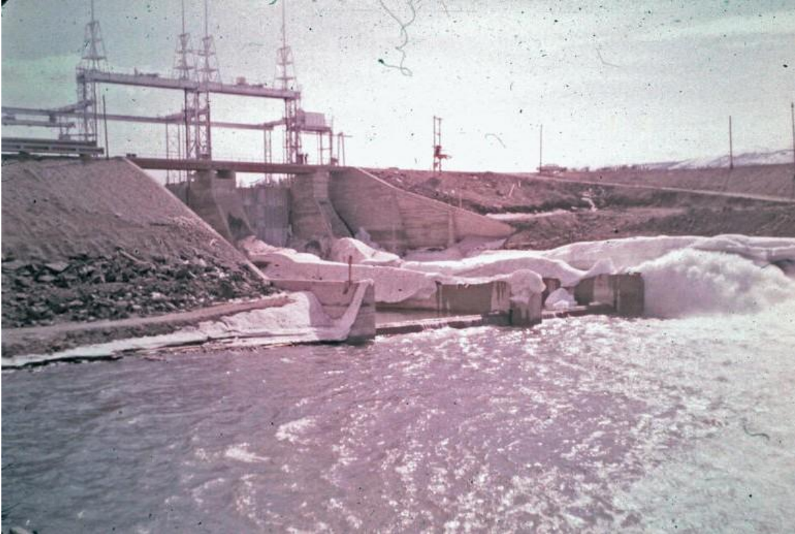
Whitehorse Dam during construction
