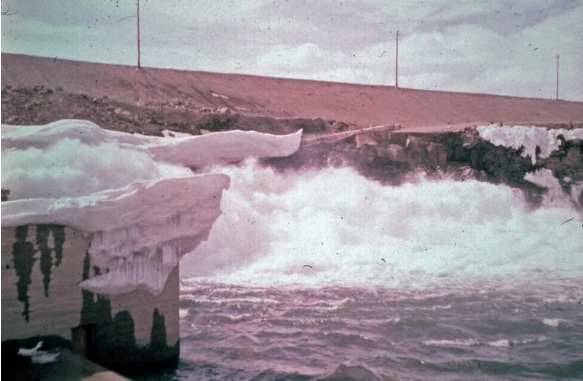
Whitehorse Dam during construction Photo courtesy Ira Saunders sandisaunders*rogers.com (In Ottawa)
