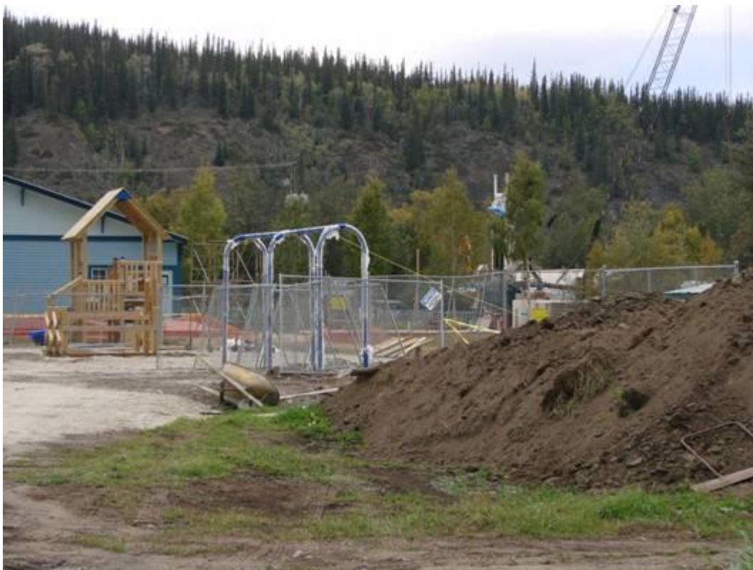
Work continues on the new playground.
