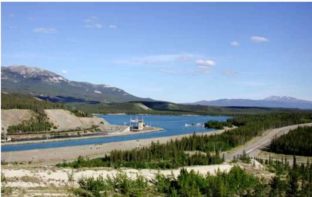
Fish ladder appears as brown wood on far side of Yukon river. Foreground is power canal that moves water from Schwatka Lake towards the intake to hydro units. Photo courtesy Tim Kinvig kinvig@northwestel.net (In Whitehorse) Sept
