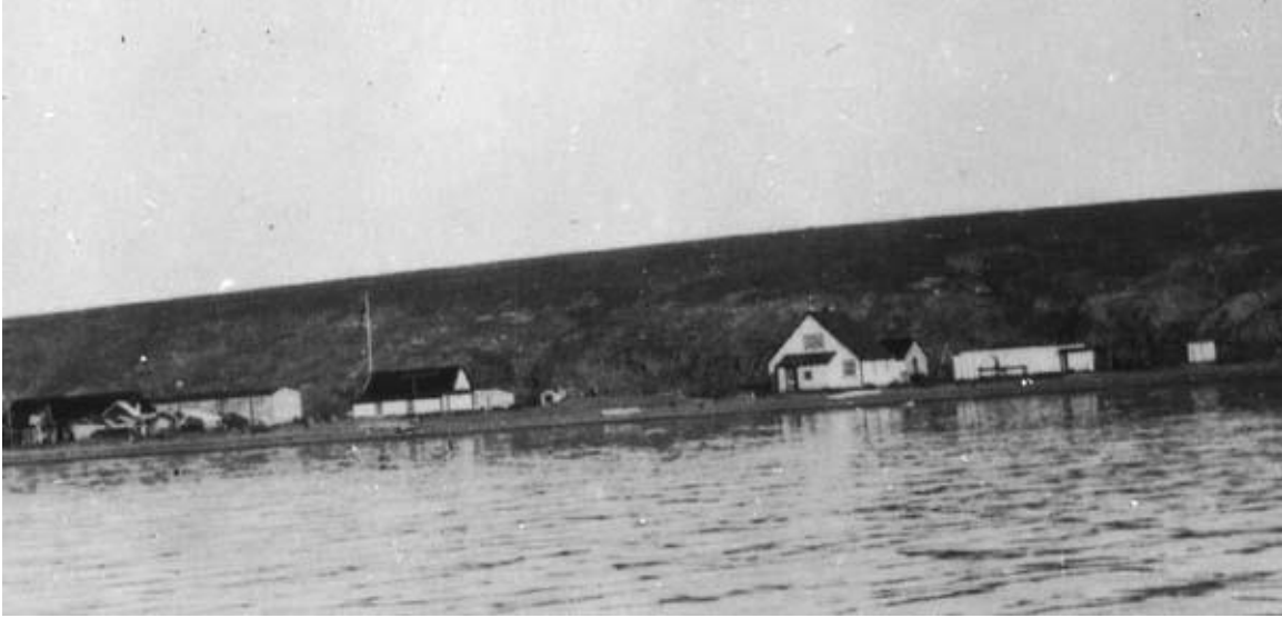
Old buildings at Herschel Island, Arctic Coast, Y.T., 1930. Yukon Archives. Finnie Family fonds, #392.
