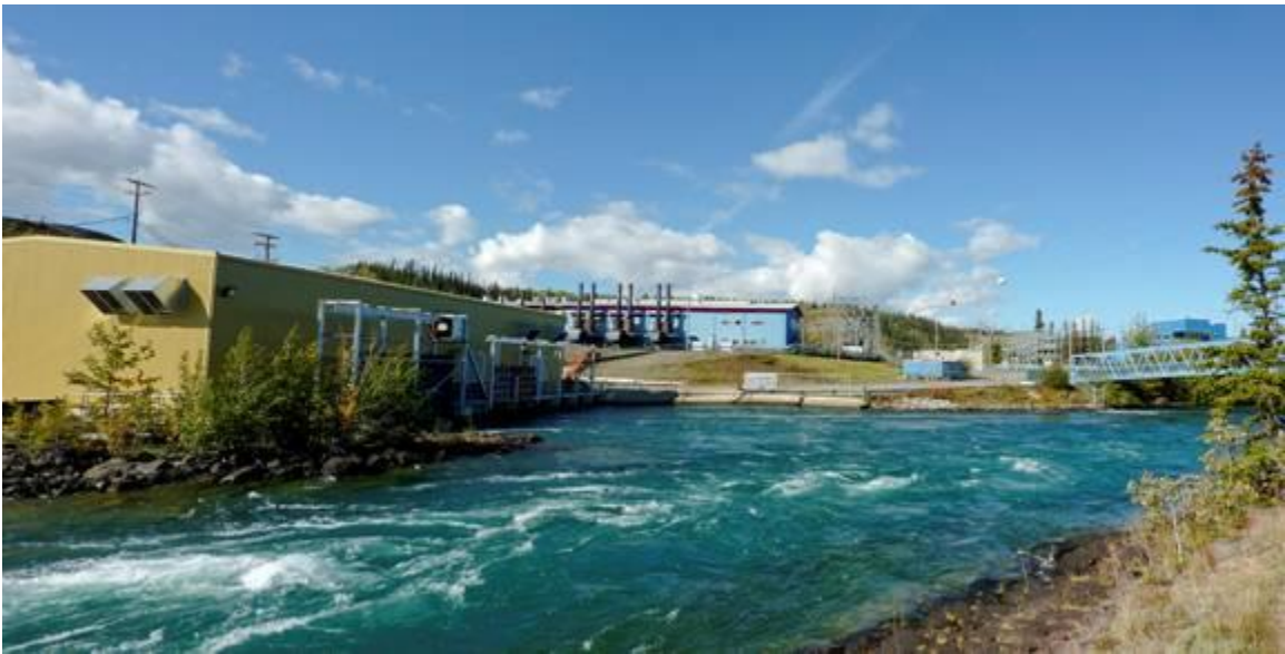
Yellow building houses Hydro Turbines # 1, 2, and 3. The blue building beyond it, houses seven backup diesel generators. Blue building far right houses Yukon Energy's corporate office. Between the two blue buildings is the substation where a voltage boost is applied to help it travel along the power lines.
