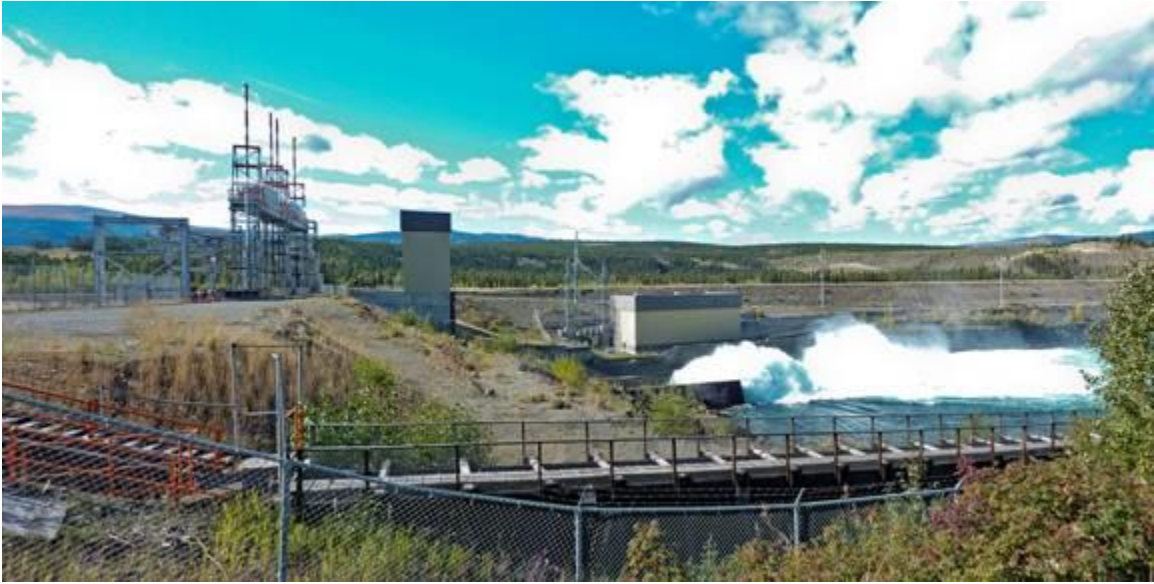
The left portion of the photo looks across the top of the Dam, and how narrow it is to consider driving across as we did back in the 1970's. Fishladder in the foreground. Yellow building beyond the spillway is Hydro turbine #4 known as the 'Fourth Wheel'.
