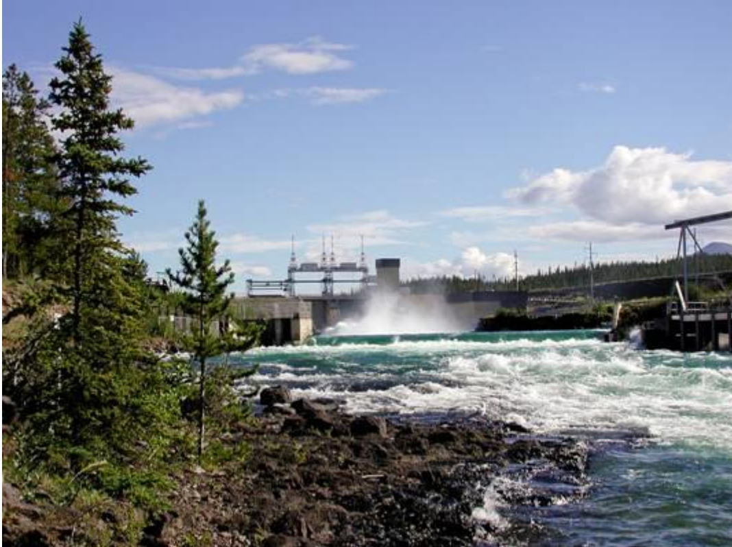
Fishladder intake on left, hydro fish screens extreme right. Spillway leaving a mist above the Fish Wier (holding back elevated water level) that directs fish towards the ladder (intake left). Photo courtesy Tim Kinvig kinvig@northwestel.net (In Whitehorse) Sept
