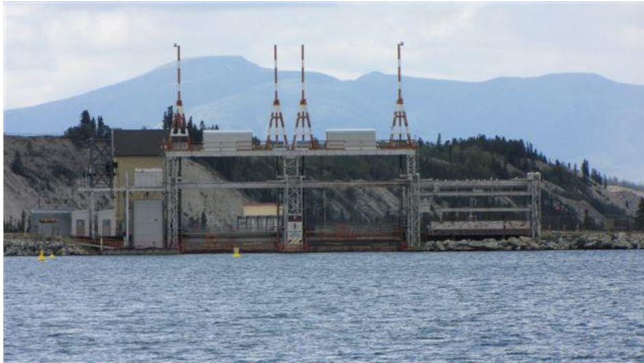
You do not see the bermed area which exists to the left of the view above.
