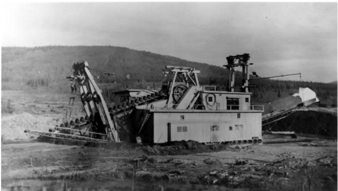
Small Dredge Working
