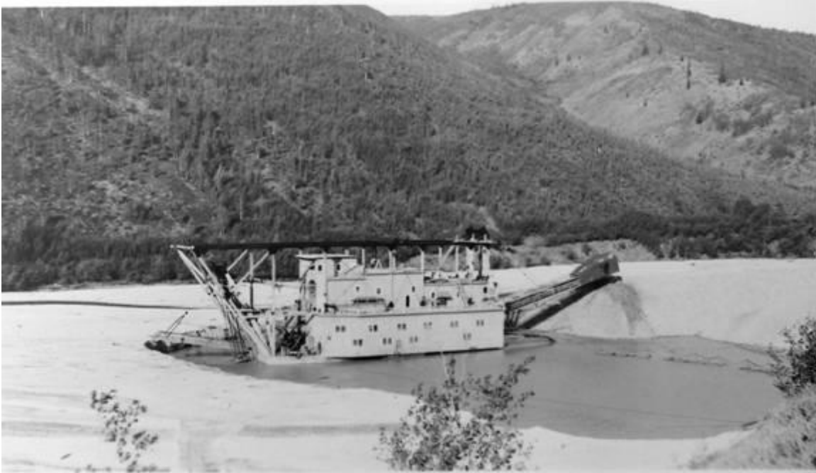
Dredge in Pond
