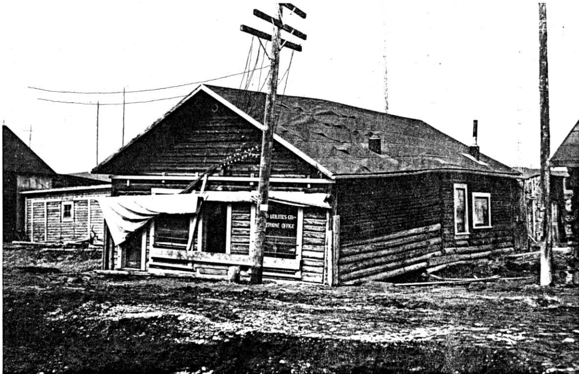
Mayo Utilities office building following the flood in 1936. Hare Collection, Yukon Archives
