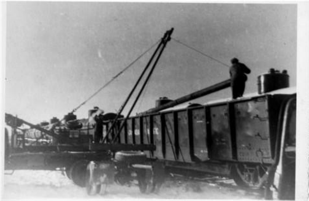
Canol Project – 1943 – Unloading Pipe Photo courtesy Donna Clayson bdclayson@northwestel.net (In Whitehorse)
