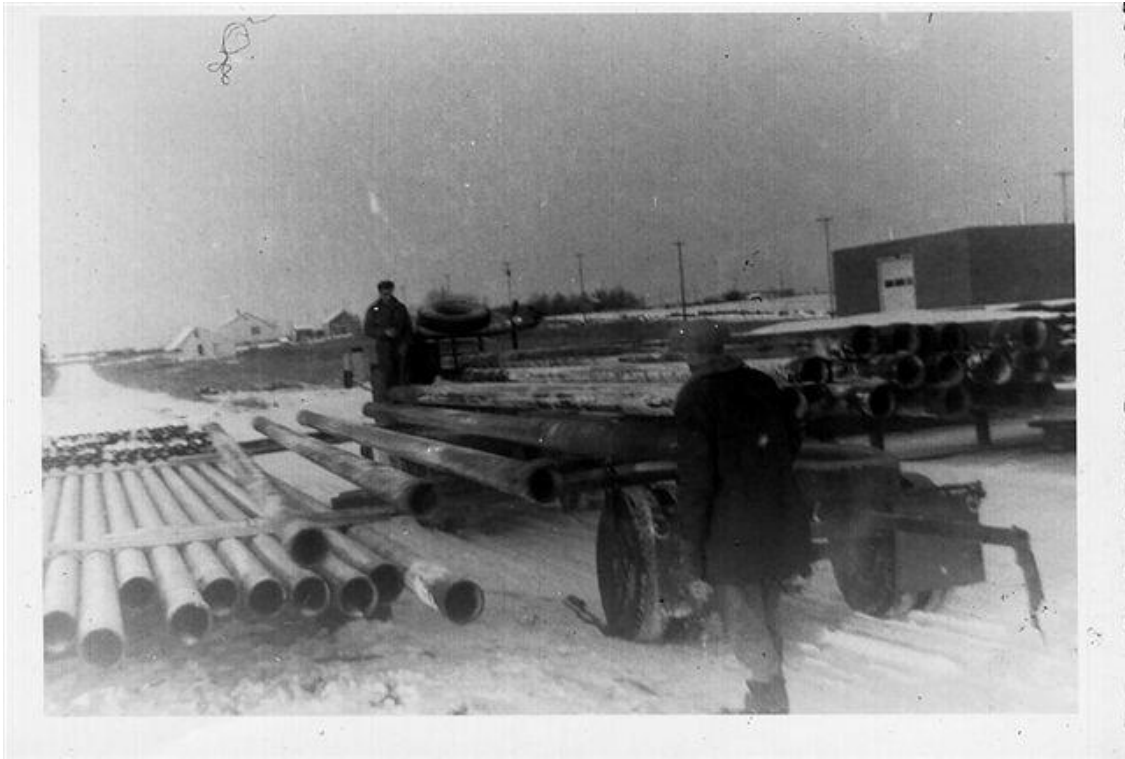
Canol Project – 1943 – Unloading Pipe Photo courtesy Donna Clayson bdclayson*northwestel.net (In Whitehorse)
