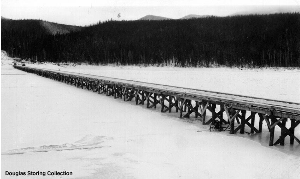
Teslin Bridge during construction of the Alaska Highway 1942-43 Photo courtesy Donna Clayson bdclayson@northwestel.net (In Whitehorse)
