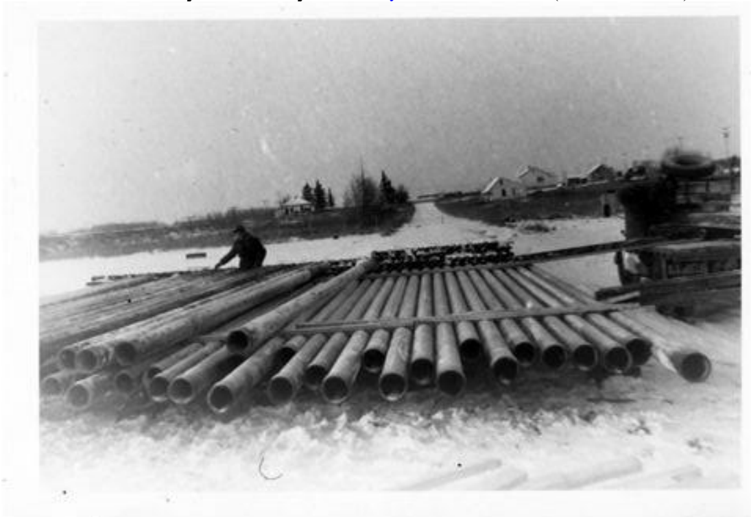
Canol Project – 1943 – Unloading Pipe Photo courtesy Donna Clayson bdclayson*northwestel.net (In Whitehorse)
