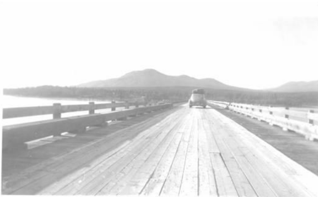
Teslin Bridge 1949 Bill Weigand bweigand@shaw.ca (In Steveston)
