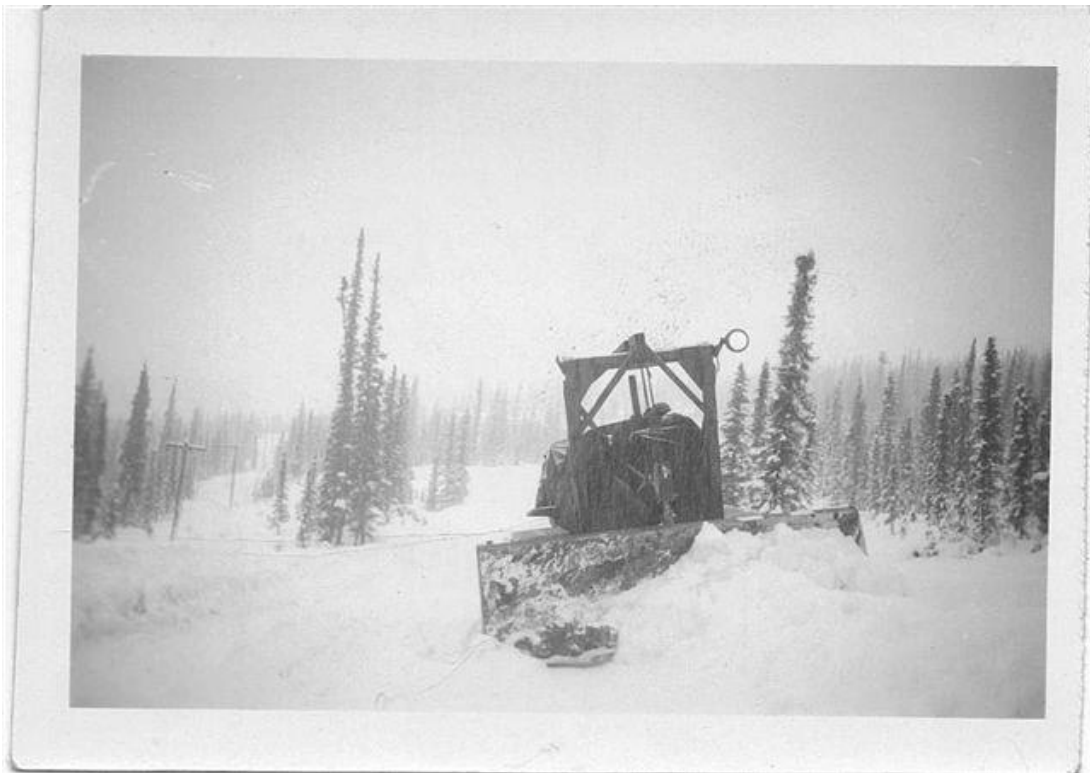
Canol Pipeline salvage project 1947-48
