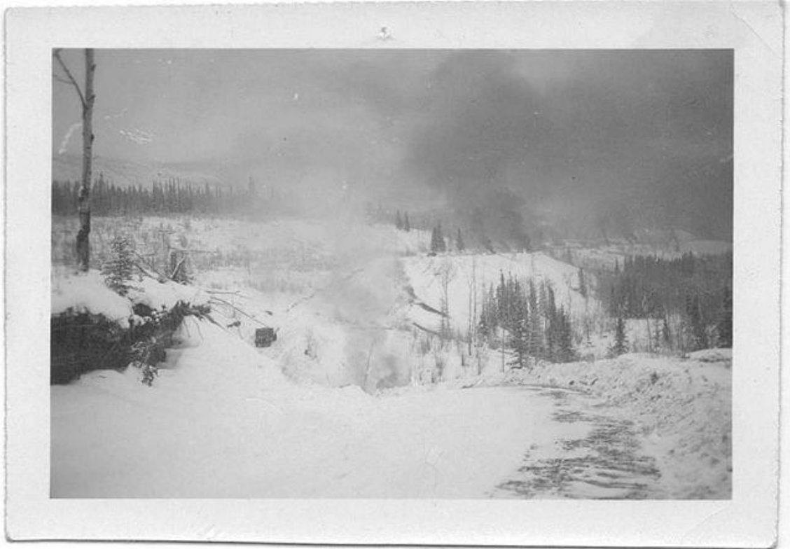
Canol Pipeline salvage project 1947-48 Photos courtesy Hal Tetz mznip@shaw.ca (In Calgary)
