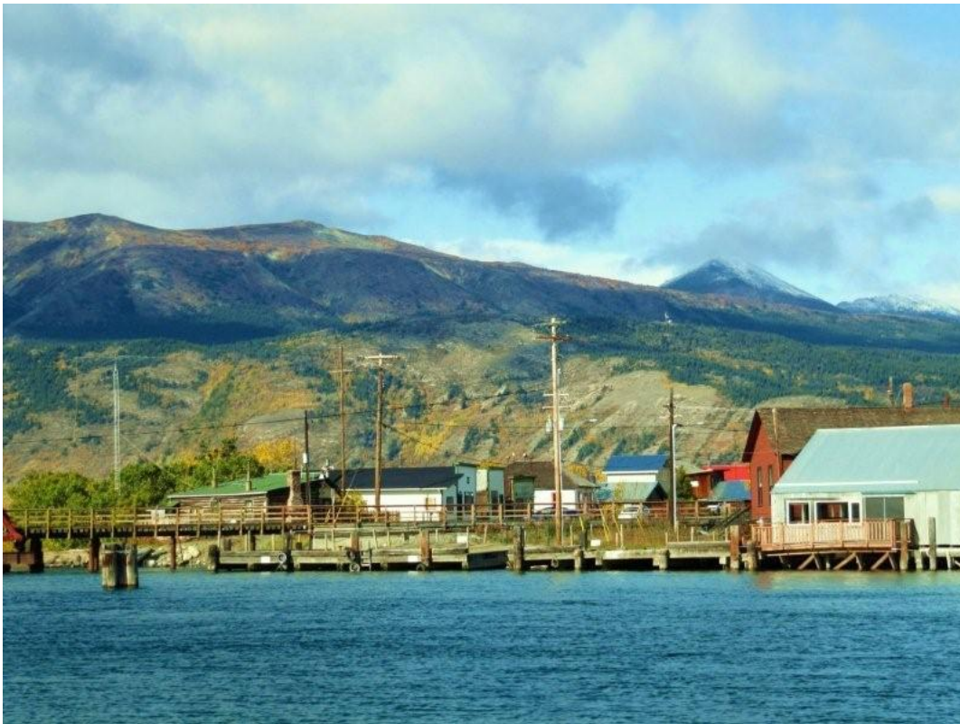
White Pass Railway bridge, wharf, and station
