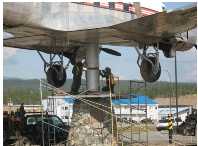
Both welders sealing the gap
