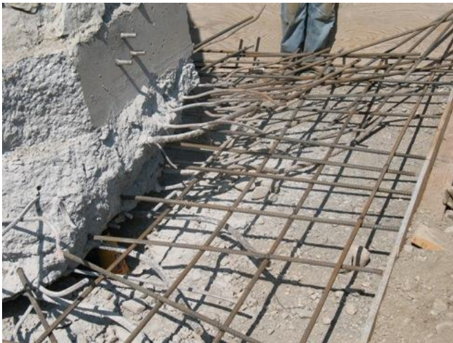
Tying in the re-bar prior to cementing
