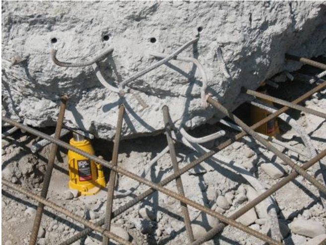
2 100-ton jacks installed on steel plates to be forever buried
