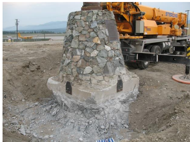
Pedestal with lifting plates waiting for flat bed truck to move it to museum site.
