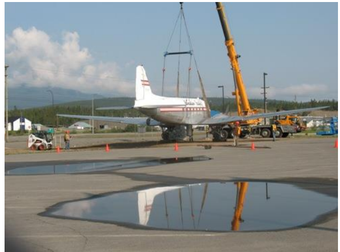
Just using the big crane with a double harness to remount CPY onto the pedestal
