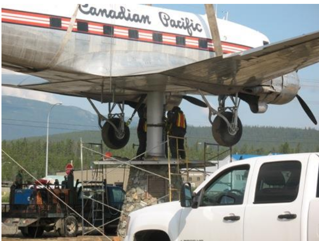
Checking for true alignment before welding seam
