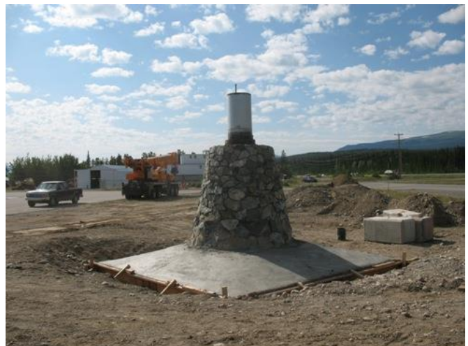
Waiting 4 days for cement to cure (looking south)
