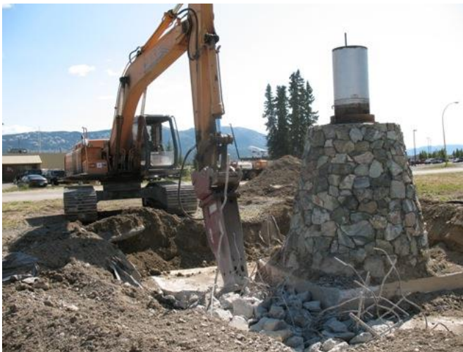
When the pedestal was uncovered a second layer 8 ft square was found and a hydraulic chisel was brought in to cut the lower base down to size
