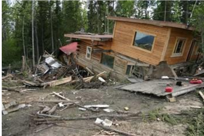
A damaged house
