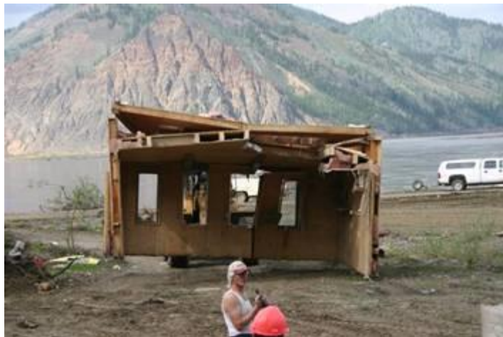
Dismantling the damage.
