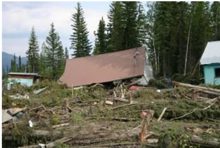
More damaged buildings
