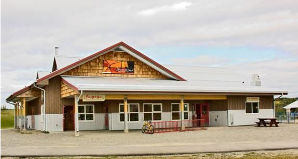
The Frank Slim Building in Whitehorse
