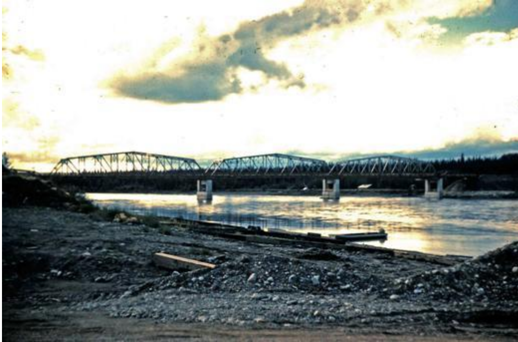
Pelly Crossing Bridge
