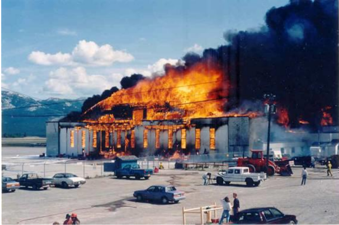
Terminal 2 or B Hangar Fire resulted from Roof Repair - July 1993 Photo courtesy Rob Austin (In Whitehorse)
