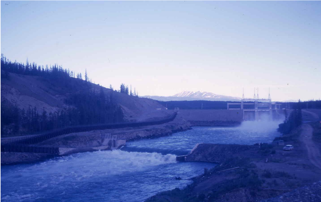
The Whitehorse power dam Note the fish ladder. Photo courtesy Emily Stillwell eistillwell@hotmail.com (Moose Jaw SK)
