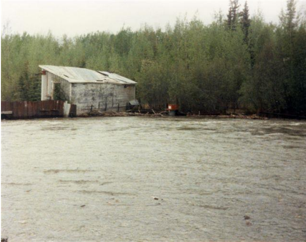
North Fork Intake
