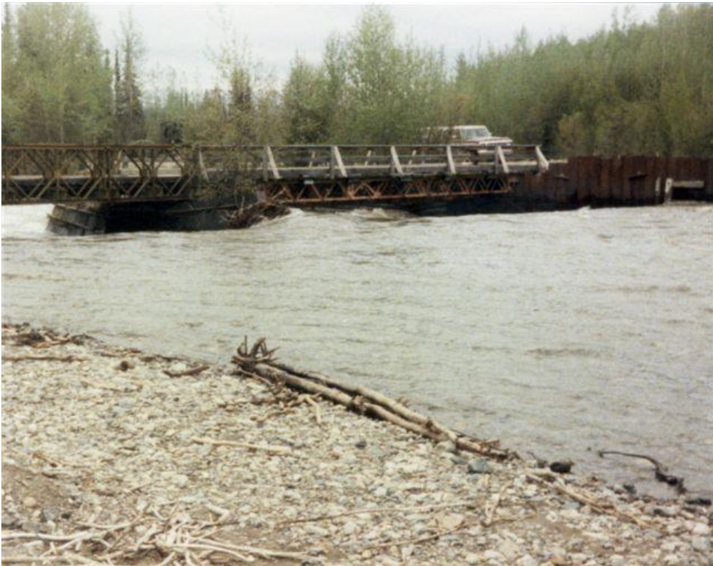
North Fork Intake
