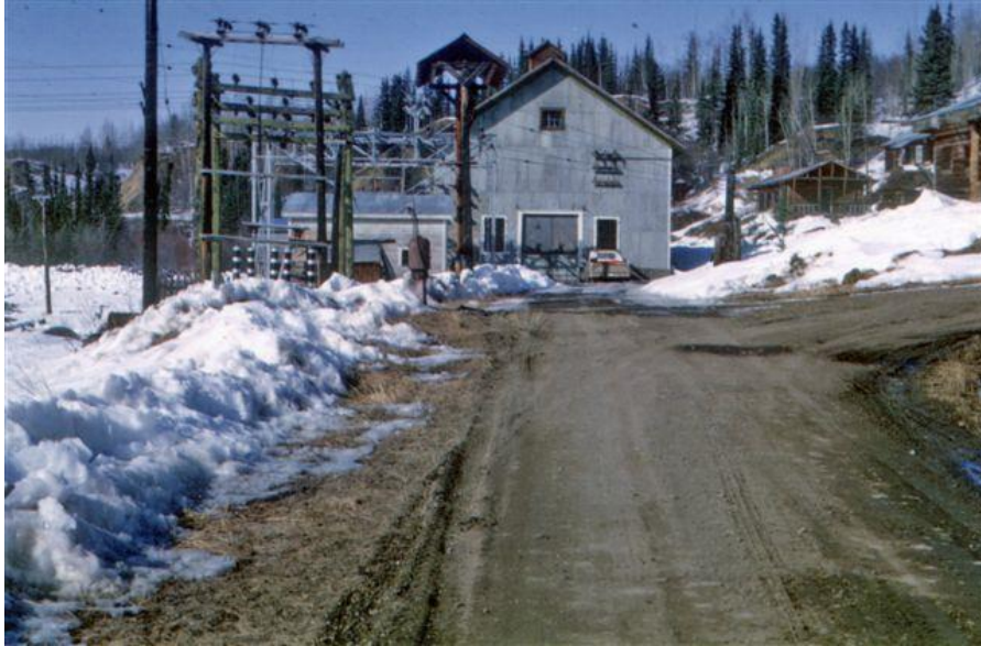
North Fork Power Plant
