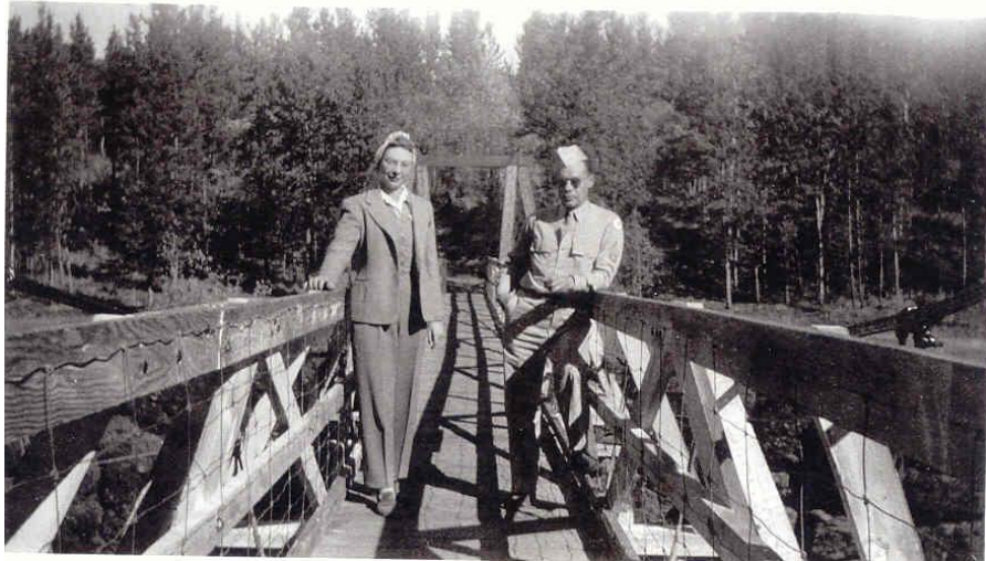
Robert Lowe Bridge – Miles Canyon
