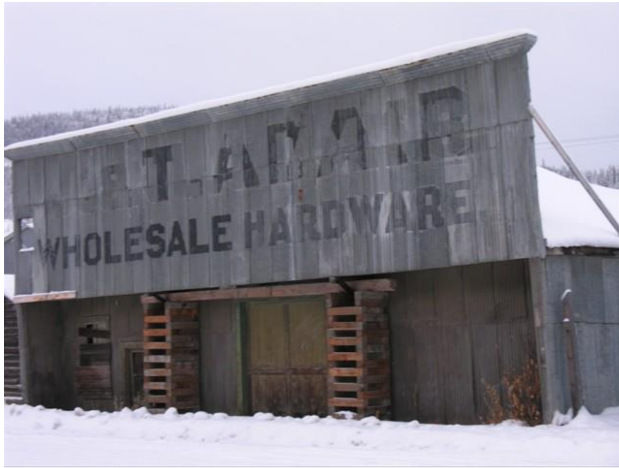
This building use to be Fred Caley's Warehouse. If anyone out there remembers, Fred Caley had probably the only neon light in Dawson, advertising his store. Photo courtesy Kris (Haydon) Janus janus*northwestel.net (In Dawson)
