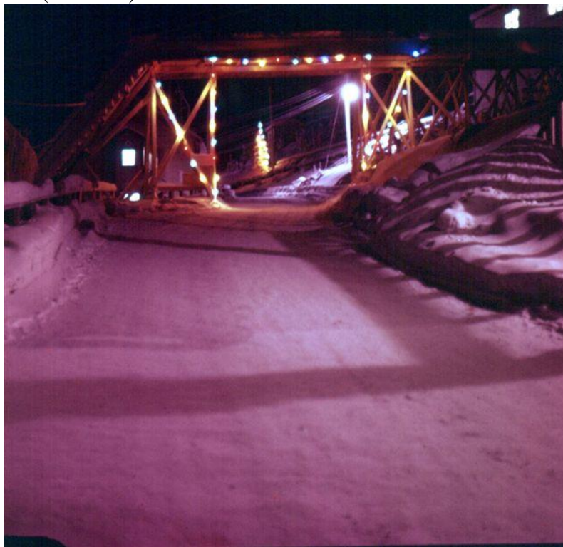
Overpass for the utilities.
