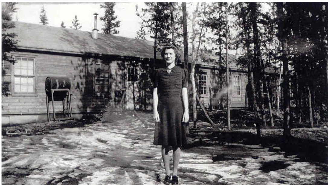
Army Building in Whitehorse - 1948
