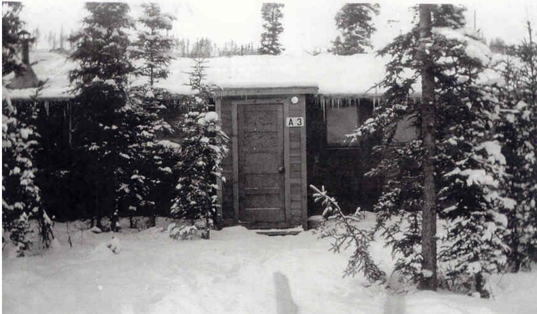
Army Building in Whitehorse – 1948
