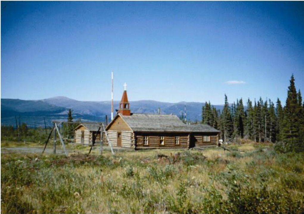
Mission school at Burwash Landing
