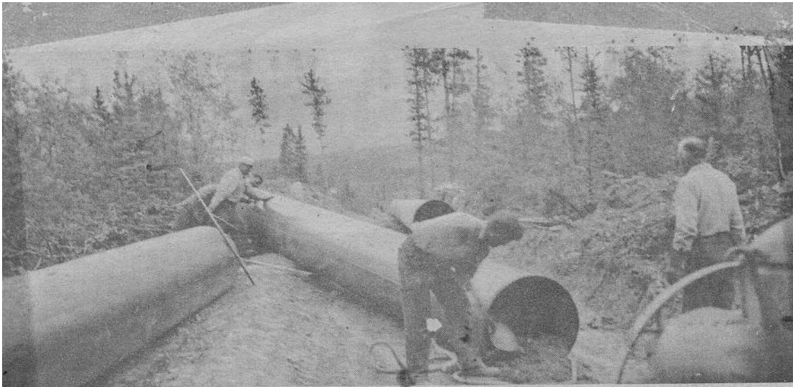
BUILDING THE HYDRO: It was in 1949 that the hydro plant was built above Whitehorse, using water from Fish and Louise lakes. John Scott and John Phelps were responsible for the
