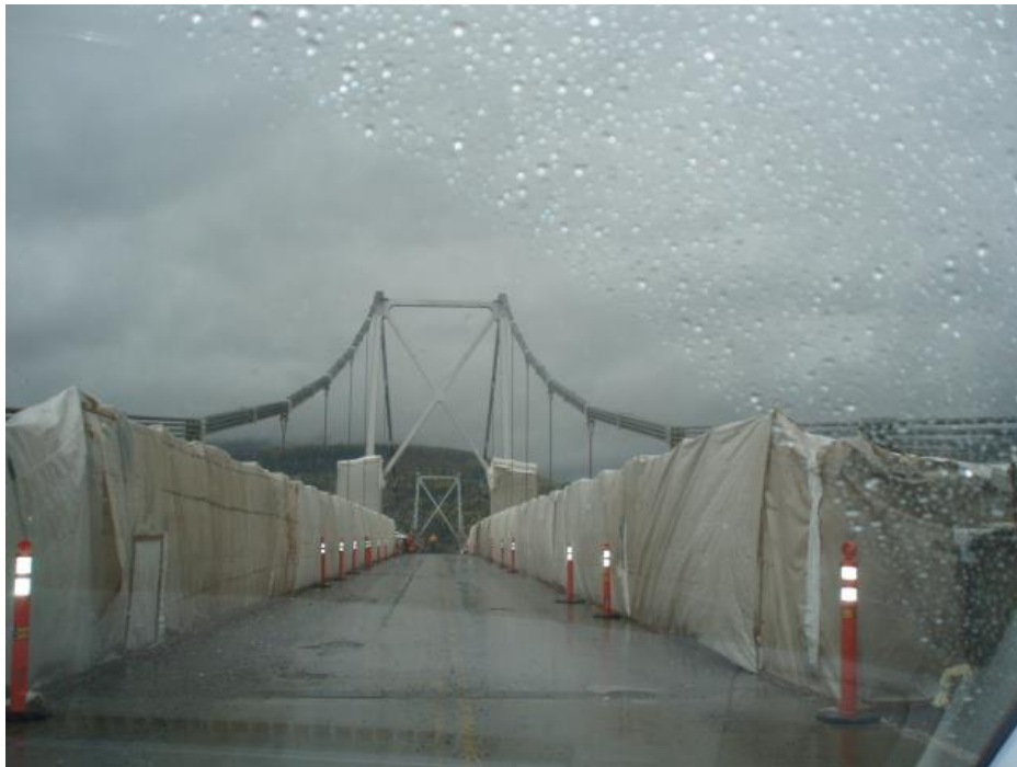
Liard River Bridge under repair – September 2007
