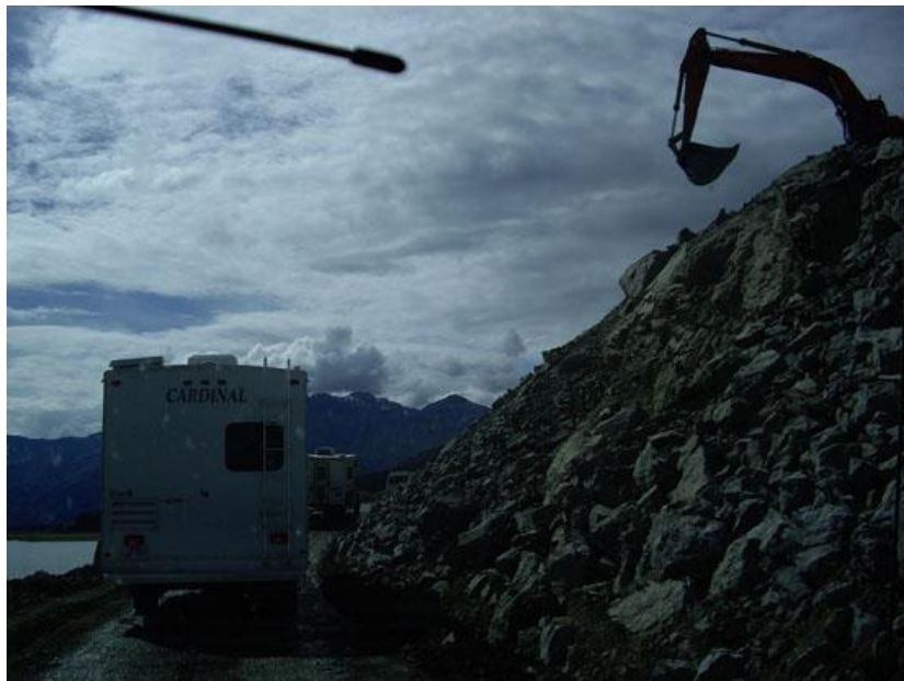
Shovels working overhead the narrow trail stop while traffic passes through.
