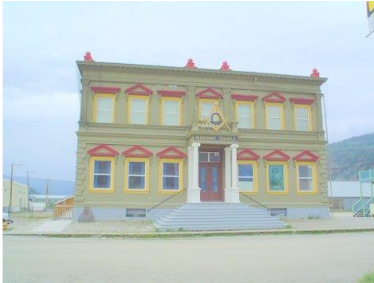
Masonic Hall after many renovations –June 2007.
