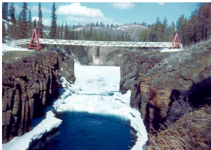
Lowe Bridge / Miles Canyon Bridge
