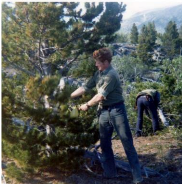
Dave Simpson from Bow Lake, Banff National Park, Alberta. He is clearing a sight line on the center line of the new road a mile or so east of Log Cabin.
