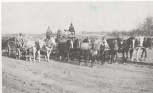
Railway construction near Wembley, Alberta. 1927. This elevating grader was powered by 18 horses, 12 pulling and 6 pushing. Brother John driving and myself standing at left on grader.
