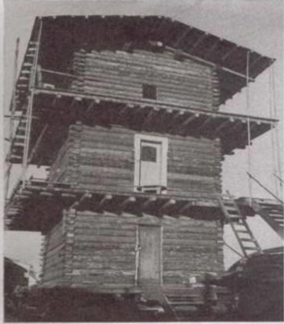
A Whitehorse "sky scraper" is this rustic "apartment house". The idea is the result of heating problems and the builder figured the stove in the lower room will heat all the floors
