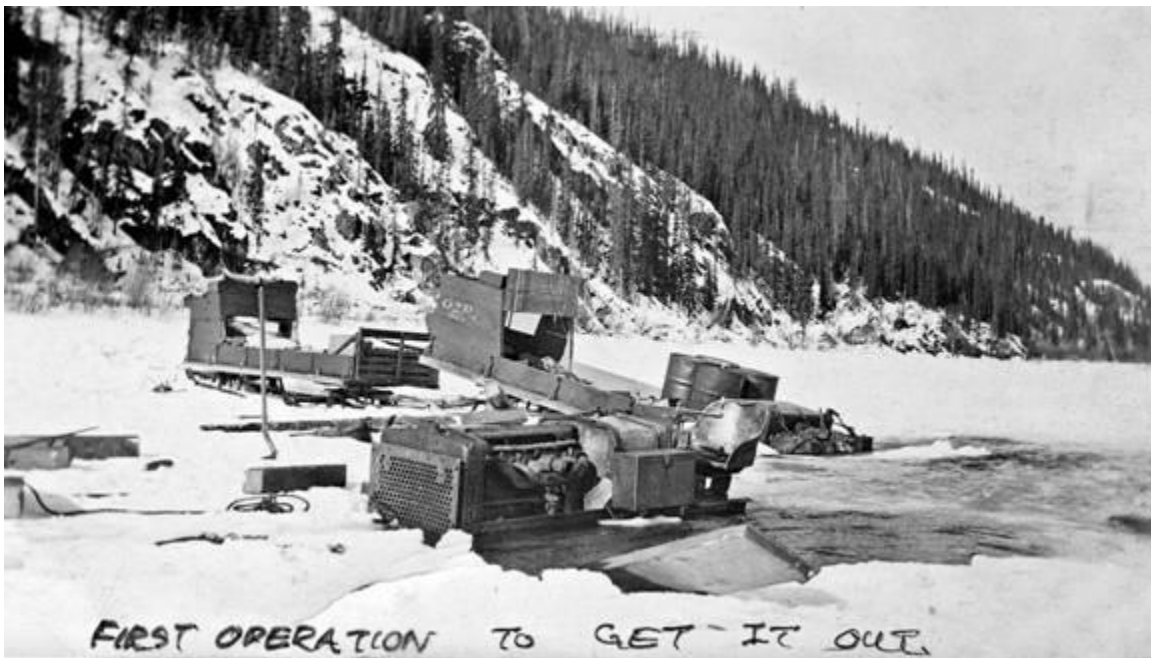
Note G & P on the side of sleigh Photo courtesy the late Les Somerton – Ernest Somerton Photo. Dawson Trail - Circa. 1926 – 1928
