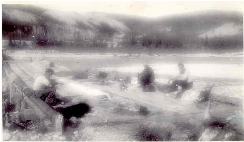
Sitting on the remains of the Little Keele River Bridge where plane found us.
