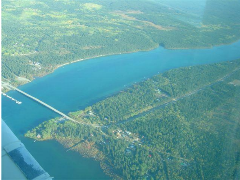
Tagish Bridge – Sept. 8 2004
