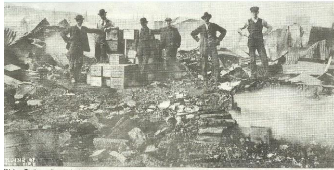
Whitehorse Fire Damage, Six men salvaging what they can, May 23, 1905 Scharschmidt Collection/Yukon Archives Photo
