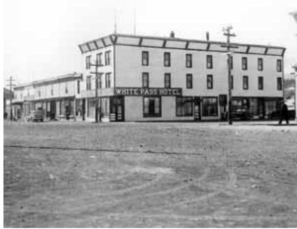
1946 Photo of the group of buildings that were destroyed in the fire. Photo courtesy Hougen Group
