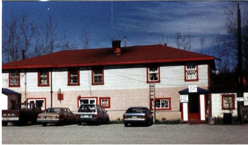
Johnson's Crossing Lodge abt 1990 Photo courtesy Aksel Porsild
