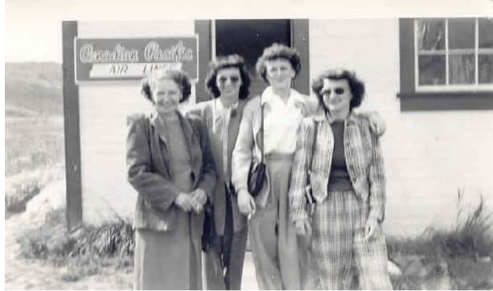
Photo Courtesy MaryAnn (Laurin) Kelleway
